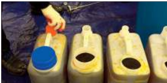
51. Seal containers air-tight. If JS comes in contact with air, it can form white crystals.
